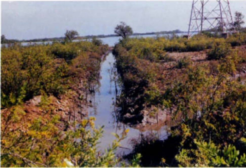
Cutting of artificial canal along the mangrove lands, for preventing the growth of salt marshes at Pichavaram
